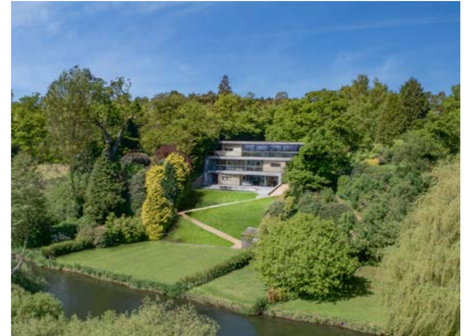
Folding House River Avon, United Kingdom Architect: Andy Ramus, AR Design Studio
